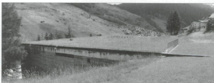
Exterior view of building showing planted roof and surrounding context. 2006. Photograph © Scott Murray.
